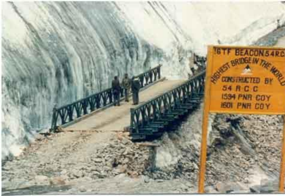
Completed 90-ft single-single Bailey Bridge
